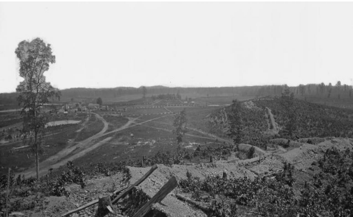
These earthworks--crucial to Johnston's defense at Resaca--were destroyed in 20th Century when I-75 swept through the heart of the battlefield. National Archives
