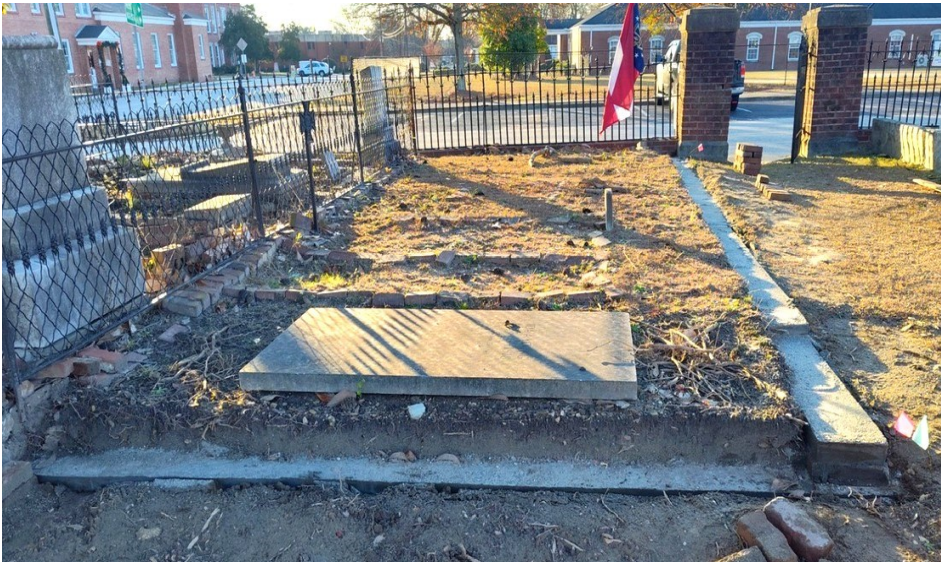
👉 While working in conjunction with the Thomson Cemetery Committee, Thomson Guards Camp 91 Compatriot Ron Awe volunteered to replace 35' of crumbled and fallen brick wall that encloses the plot of a Confederate soldier. Mr. Epp Wilson's fence crew removed the old structure and Compatriots David Moore and Tom Holley cleaned most of the old bricks. Ron poured the concrete foundation and replaced the wall. Because the committee receives no financial support from the county or city for the cemetery, Camp 91's volunteer work has been essential to returning the cemetery to its former glory.
