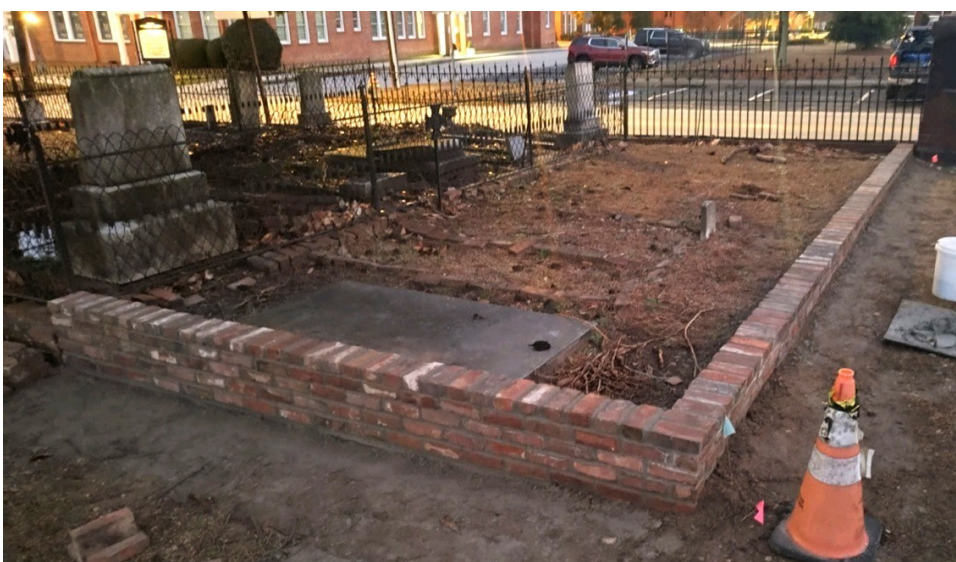
👉 While working in conjunction with the Thomson Cemetery Committee, Thomson Guards Camp 91 Compatriot Ron Awe volunteered to replace 35' of crumbled and fallen brick wall that encloses the plot of a Confederate soldier. Mr. Epp Wilson's fence crew removed the old structure and Compatriots David Moore and Tom Holley cleaned most of the old bricks. Ron poured the concrete foundation and replaced the wall. Because the committee receives no financial support from the county or city for the cemetery, Camp 91's volunteer work has been essential to returning the cemetery to its former glory.
