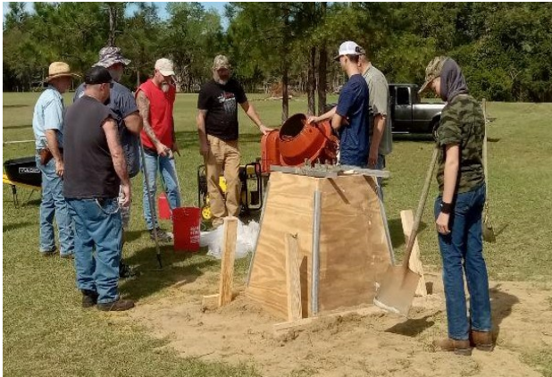
Montgomery County Sharpshooters SCV Camp #2164 and Pine Barrens Vols. SCV Camp #2039 to construct the formwork and pour the concrete base for the 50ft Flag Pole off Hwy 441 Wheeler County, Ga.
