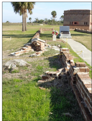
☞ L. Damage to Cemetery wall at Ft. Pulaski by last year's tornado. ☞ R. Repairs were made by Randall Burkhart, Jeffery Marlow, Jesse Perry, and the staff of the NPS.
