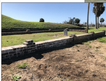
☞ L. Damage to Cemetery wall at Ft. Pulaski by last year's tornado. ☞ R. Repairs were made by Randall Burkhart, Jeffery Marlow, Jesse Perry, and the staff of the NPS.
